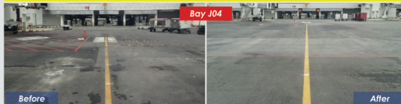
Bay J04 free from water ponding after the completion of grouting injection works.
