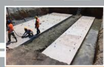
**Solution** - Installing precast concrete slab to reduce the impact of differential settlement.
