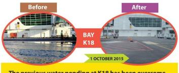
The previous water ponding at K18 has been overcome by full overlaying works.
