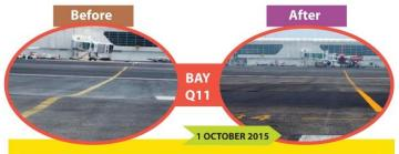
Differential settlement at Q11 has been resolved by the installation of precast concrete slab.
